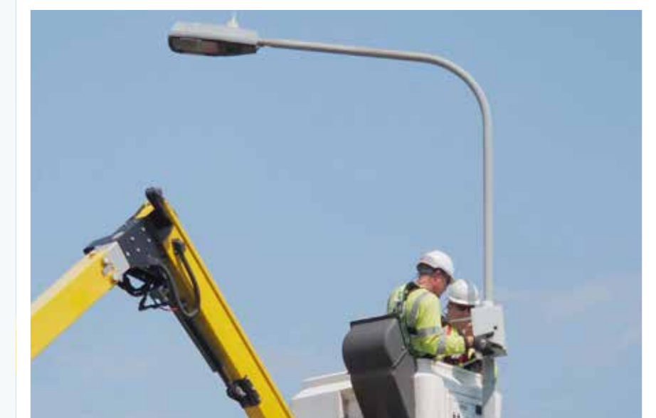
Sustainable street lighting →
